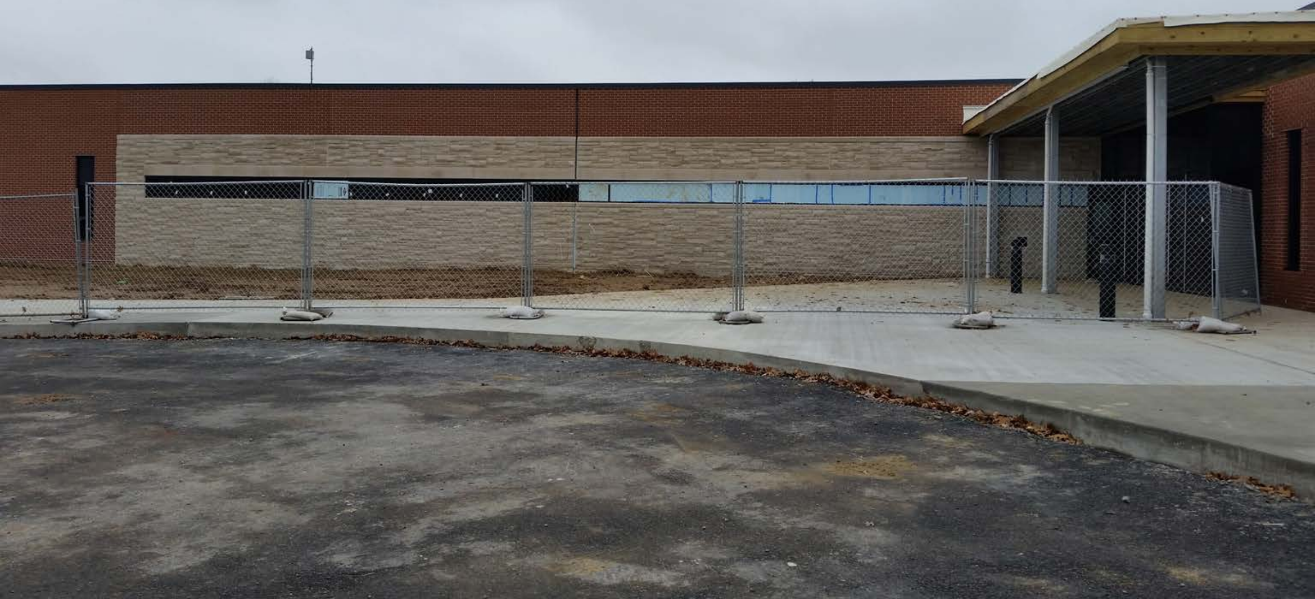
The new office wing and old lobby entrance.
